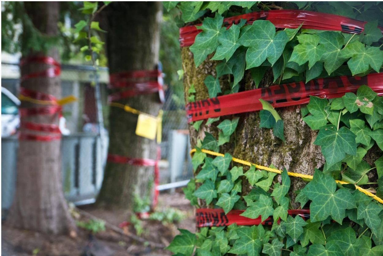
Red tape protecting trees in a construction zone
